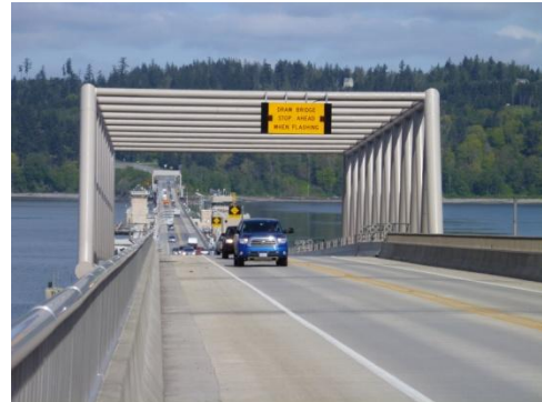
Hood Canal Bridge
