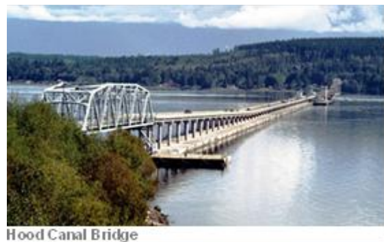
Hood Canal Bridge
